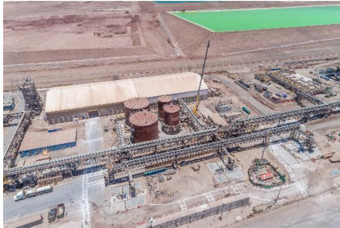
Lithium plant general view
