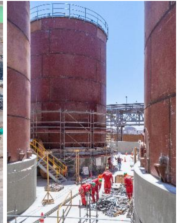
Tanks (Civil Works, Construction & Assembly)
