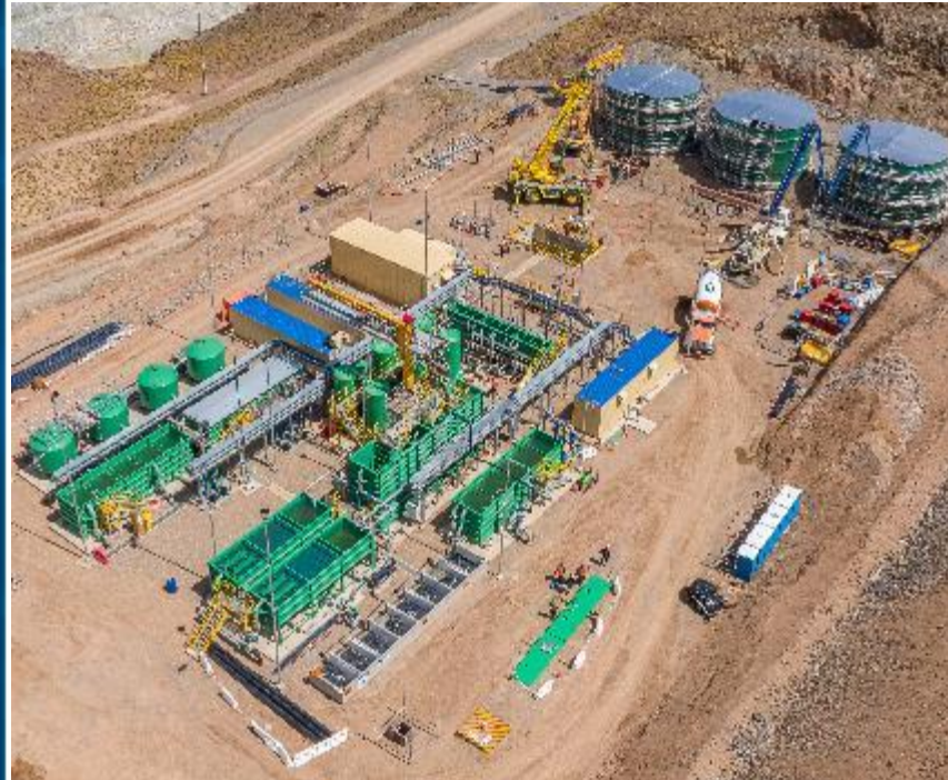
Water treatment plant general view
