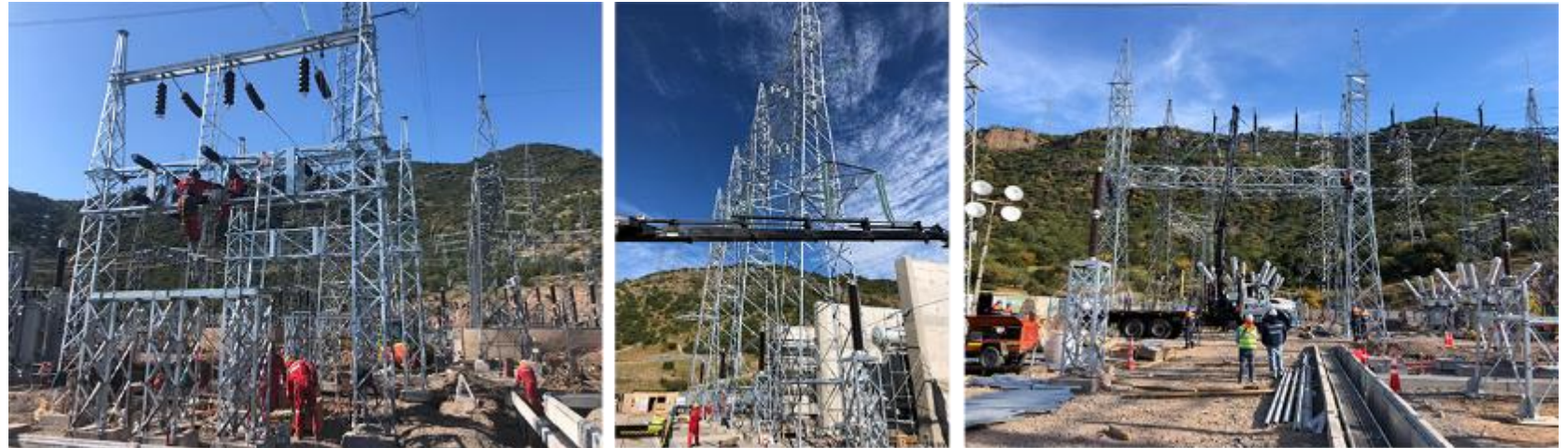
Electrical Substation general views
