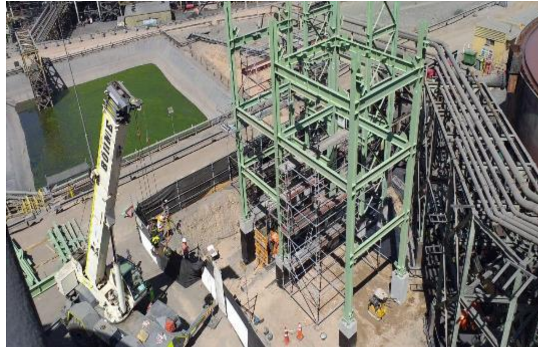
Safety Structure Assembly
