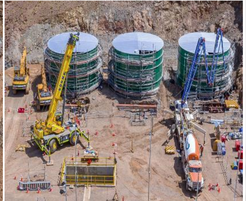
Concrete pouring for Storage Tanks
