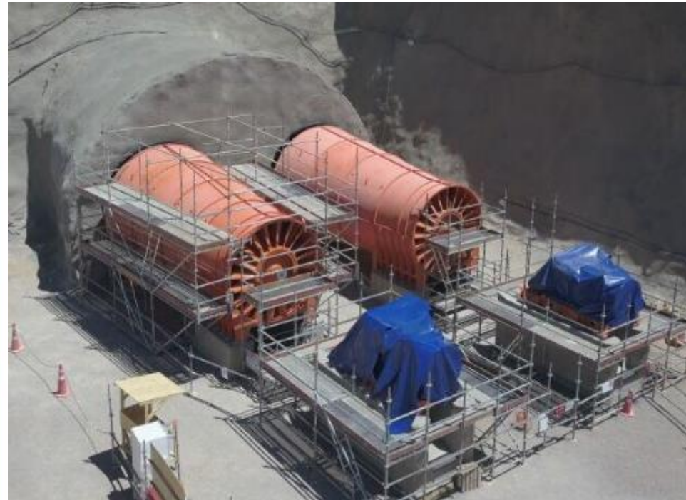
Exterior Mine Ventilators (2)
